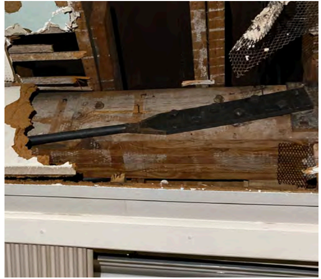
Exposed strap at timber girder Level 2
