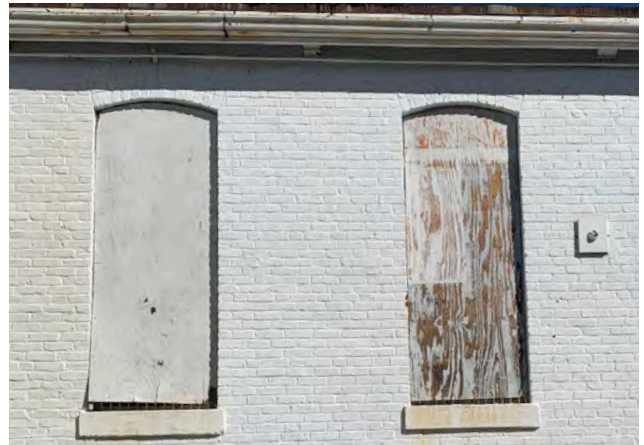
Typical widow with rowlock brick arch and limestone sill
