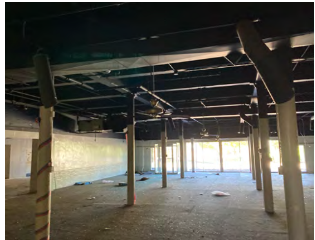
Typical 8" Timber Columns
