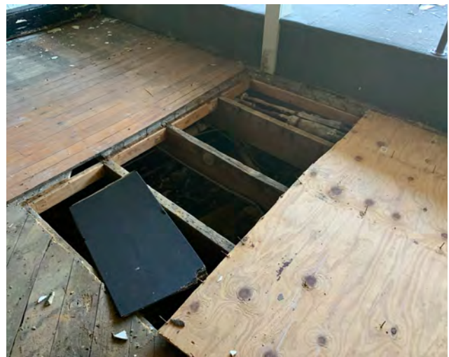
Typical Lower Level Floor Construction
