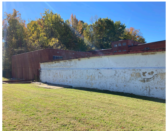
Covered Clear Well and Pumping Room with access at grade.
