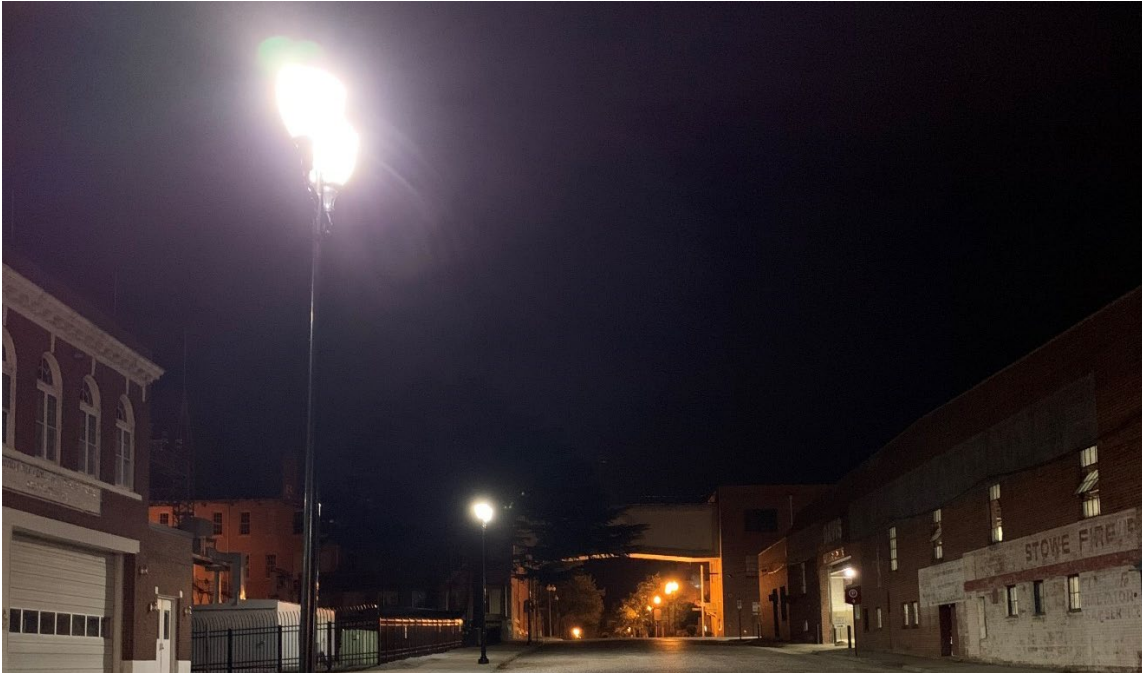
Image 9: An example of brighter replacement luminaires within a Sternberg “Danville Fixture” streetlight along Bridge Street Image Credit: RHI
