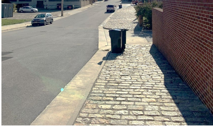
Image 2: Recent rehabilitation of an historic sidewalk along Lynn Street Image Credit: RHI
