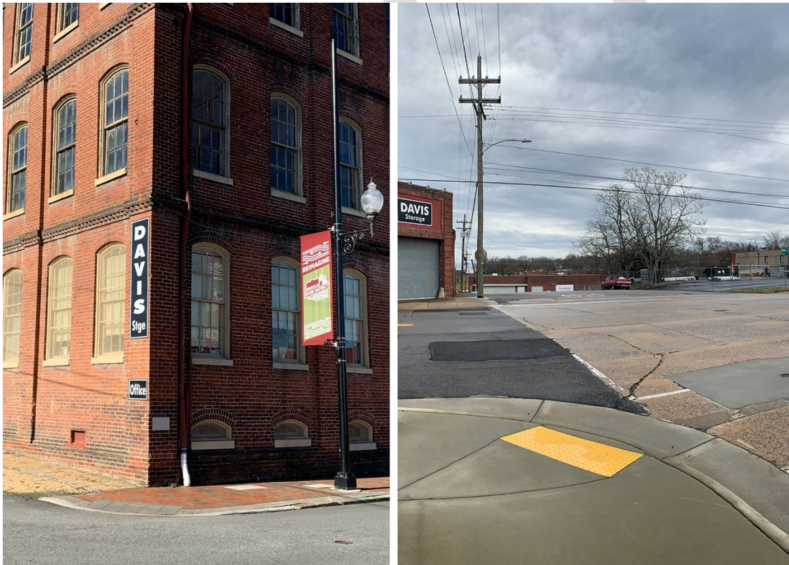
Image 3: New ADA Compliant Curb Ramps on Craghead Street (left) and Court Street (right). These curb ramps are built correctly, yet their adjoining crosswalks lack visibility
