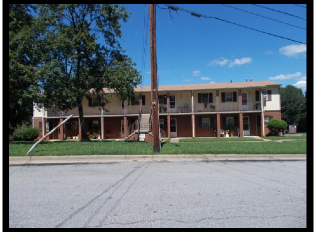
56) POPLAR STREET/UPPER STREET
